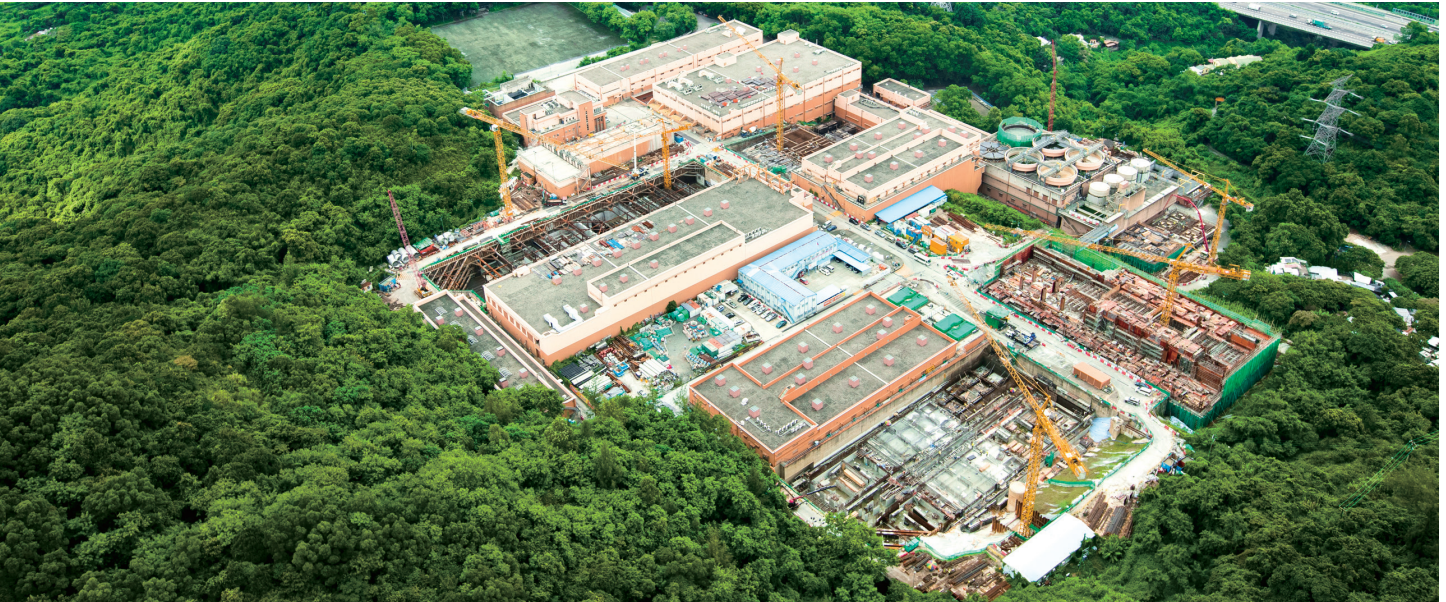
大埔濾水廠 Tai Po Water Treatment Works
