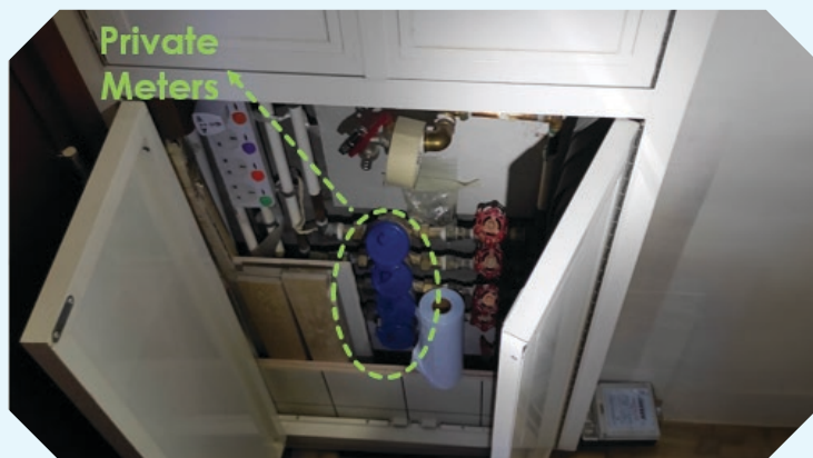
安裝水務署水錶前 Before Installation of WSD's Water Meters
