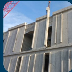
Installation of DfMA concrete wall panels onto the Product Water Pumping Station
