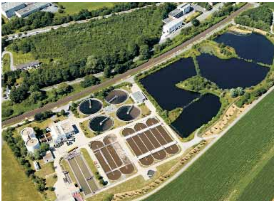
Wastewater Treatment Plant, Arnsberg-Neheim, Germany
