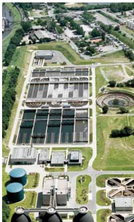
Wastewater Treatment Plant, Duisburg-Kasslerfeld, Germany
