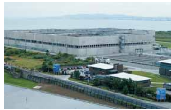
Dublin Wastewater Treatment Plant
